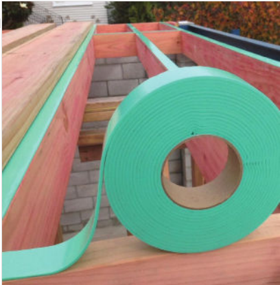
NORTON CST™ applied to wooden floor joists
